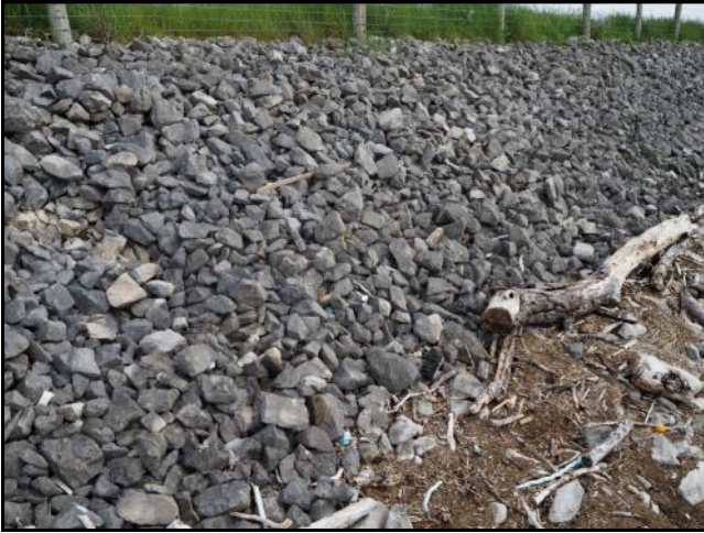
Figure 2. Stone embankment. © Chris Workman.
